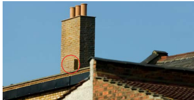
Good example of disguised equipment
