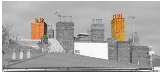
Good example of equipment disguised within existing structures Photographs courtesy of Dynamic Concepts
