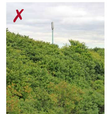
Bad example of monopole location
