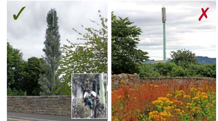
Good example of disguised equipment
