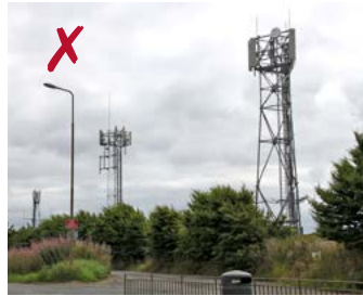
Good and bad examples of lattice mast location
