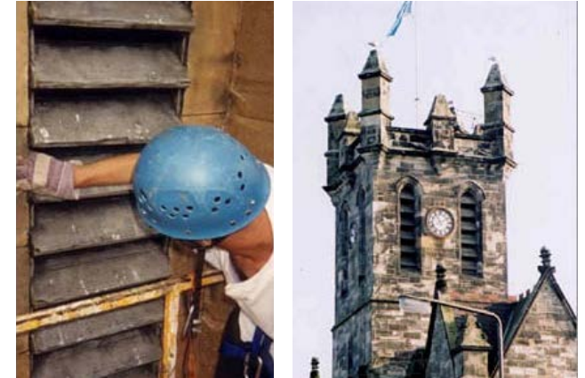
Louvre replaced on a listed building with radio transparent replica Photographs courtesy of Dynamic Concepts
