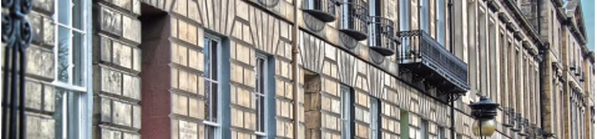
Photograph 2: New Town terrace details. Copyright CEC.
