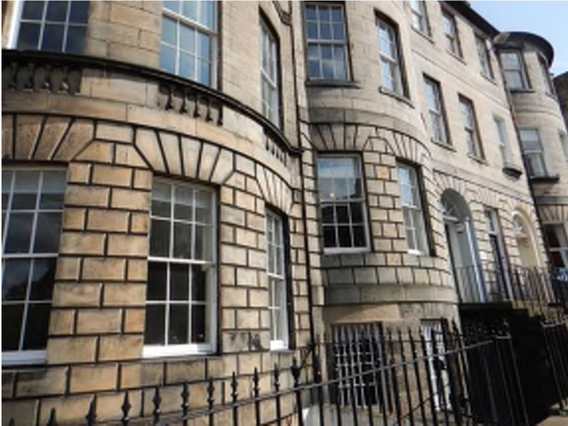
Photograph 1: New Town terrace details, circa 1795, droved cream ashlar-faced sandstone with polished dressings. Taken from the W.
