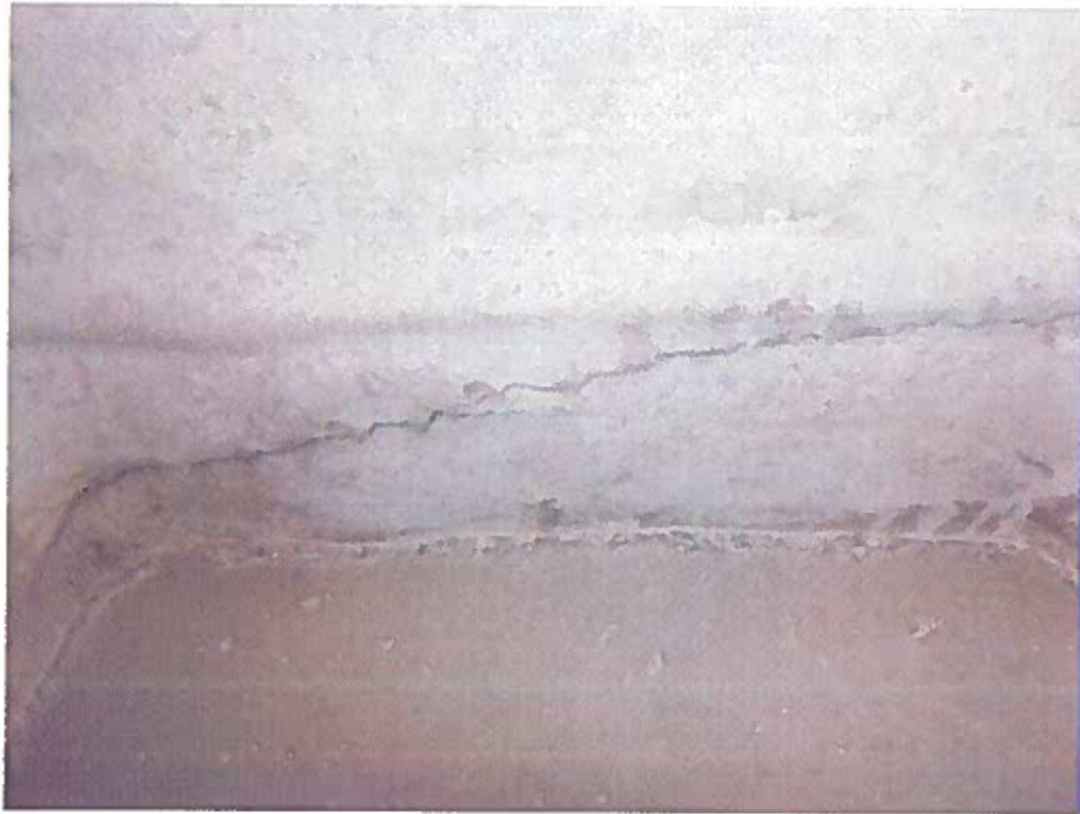
Area 2, Soffit of Slab Close Up of Crack
