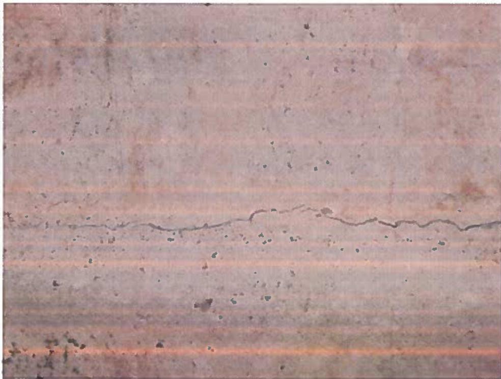
Area 1, Soffit of Slab Close Up of Crack
