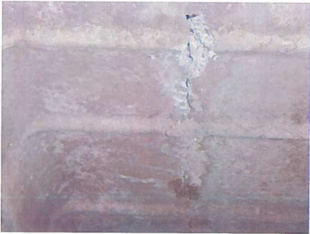
Area 2, Soffit of Slab General View Exhibiting Cracking
