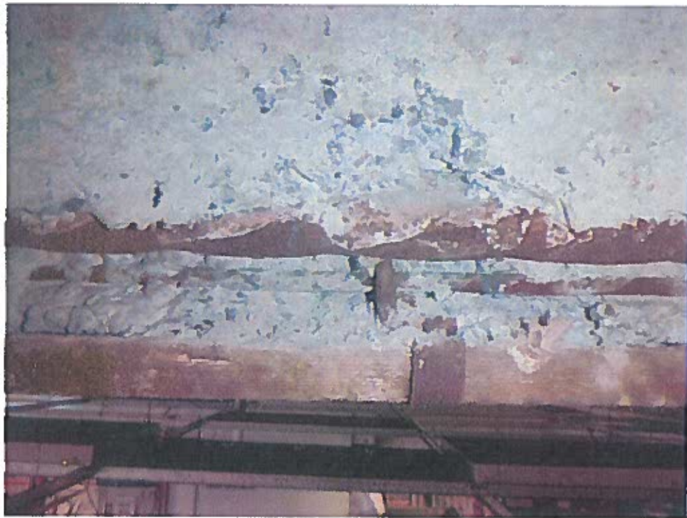
Plate 16. Area 1, Rib Concrete Cover Removed to Expose Reinforcement
