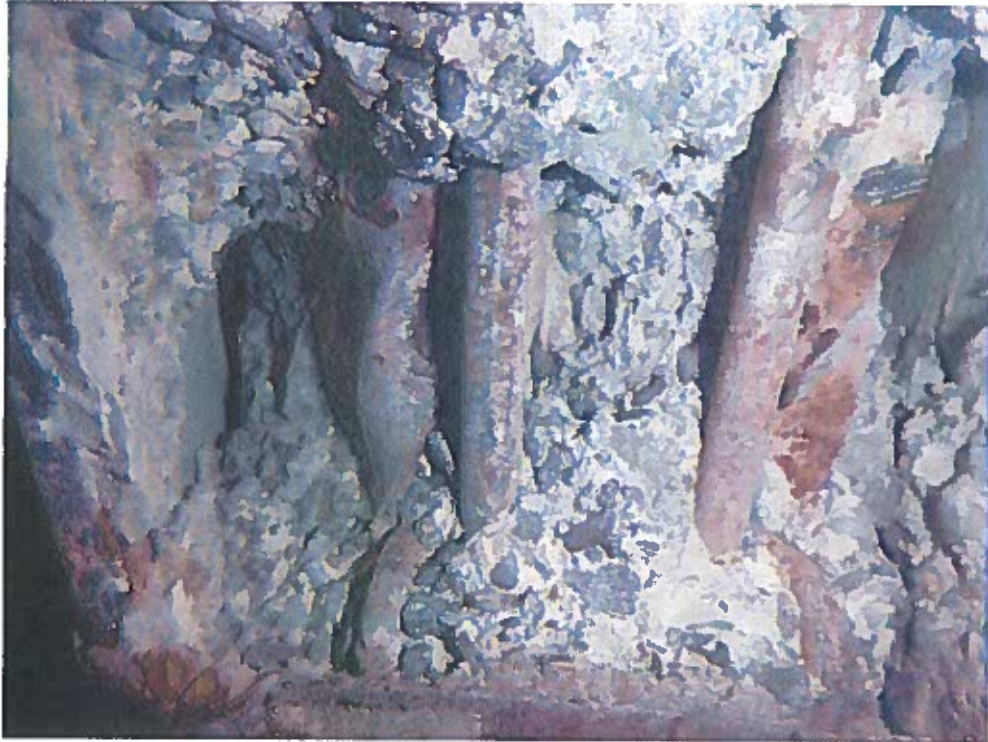
Plate 44. Area 4, Rib Concrete Cover Removed to Expose Reinforcement
