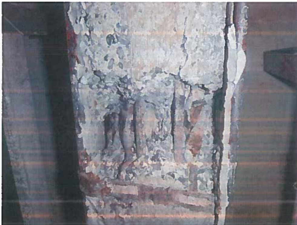
Area 4, Rib Details of Reinforcement
