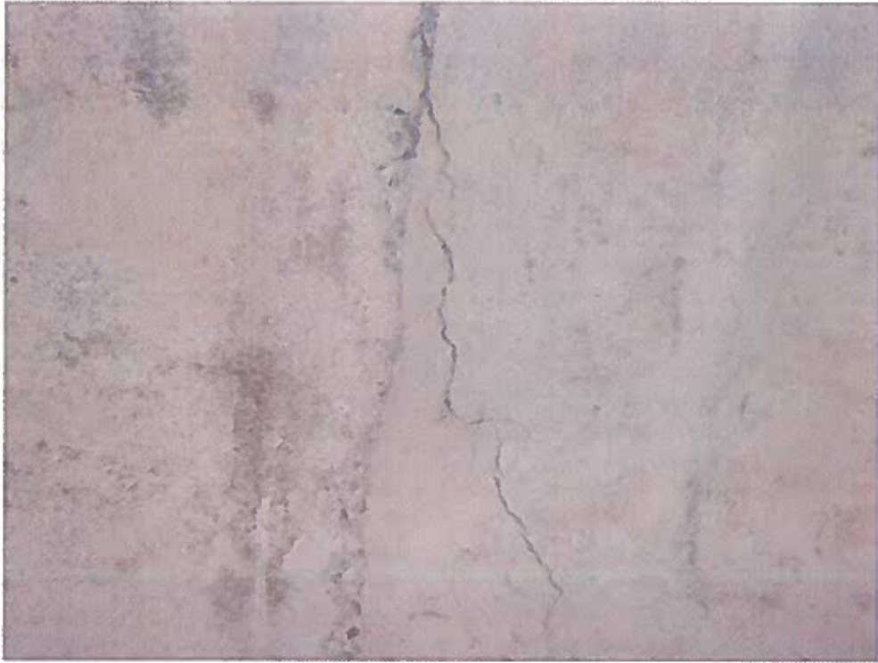
Area 1, Soffit of Slab Close Up of Crack
