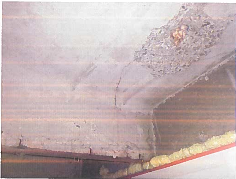
Area 2, Soffit of Slab Large Area of Spalled Concrete Due to Service Access and Adjacent Crack
