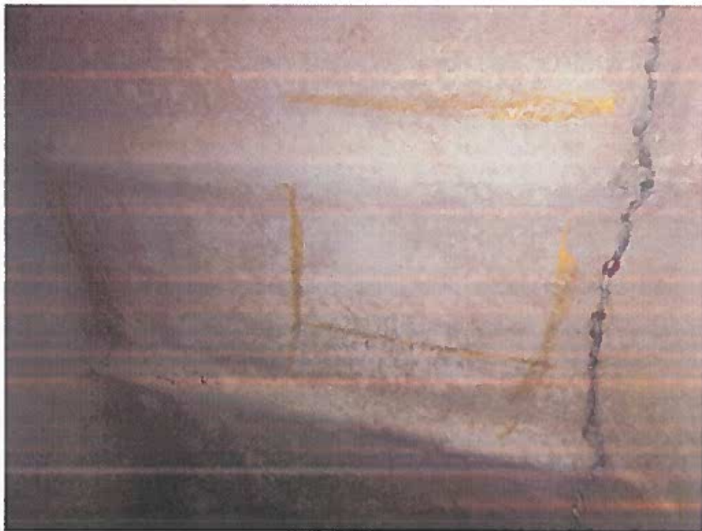
Area 3, Soffit of Slab Close Up of Crack
