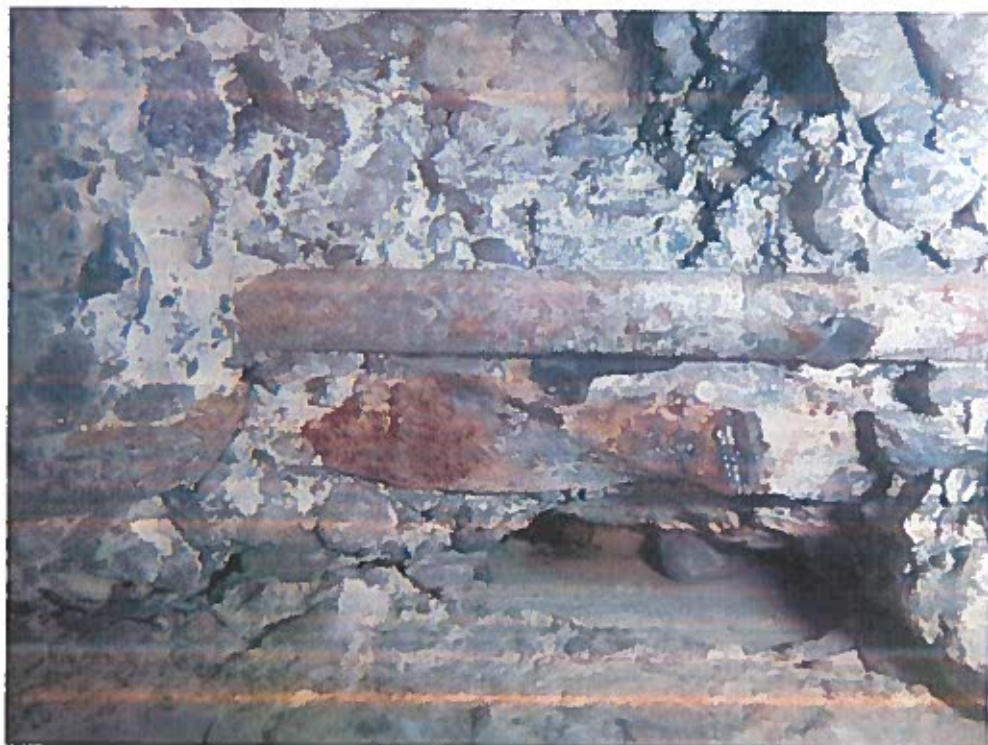
Plate 45. Area 4, Rib Concrete Cover Removed to Expose Reinforcement
