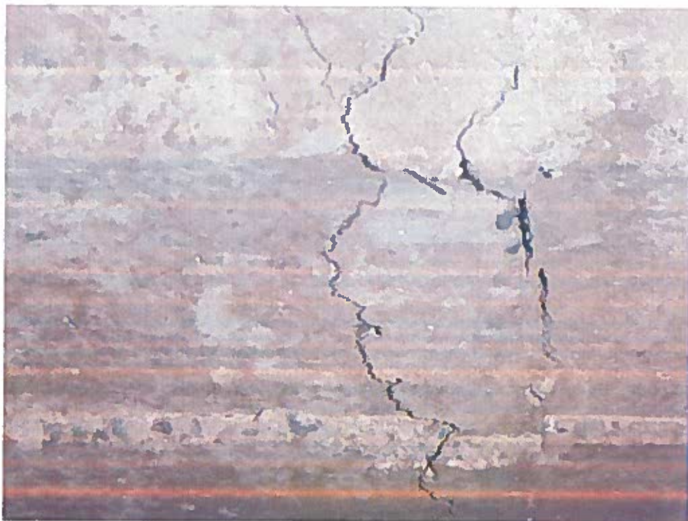
Area 2, Soffit of Slab Close Up of Crack
