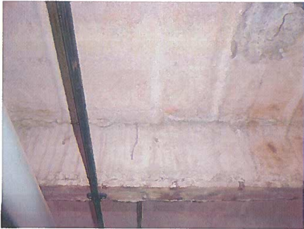
Area 1, Soffit of Slab General View Exhibiting Cracking
