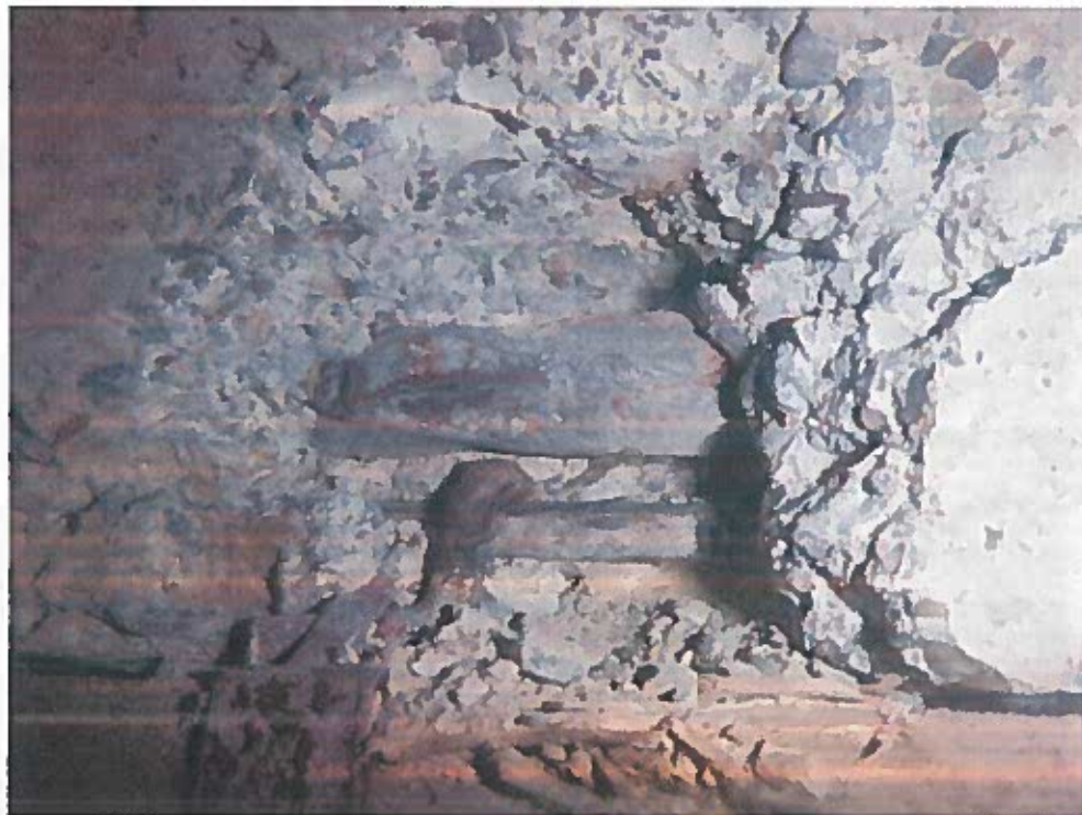
Area 1, Rib Concrete Cover Removed to Expose Reinforcement
