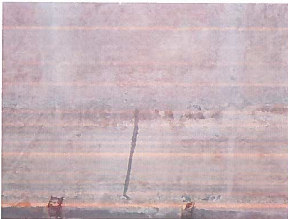
Area 1, Soffit of Slab General View Exhibiting Cracking
