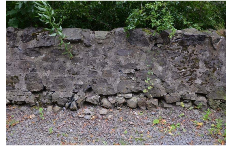
Rubble Wall on Regent Walk
