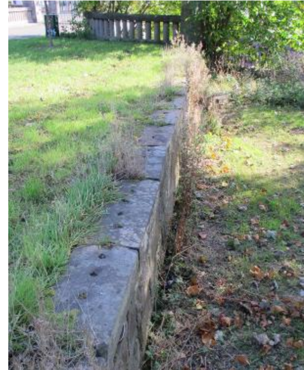
Original railing remnants
