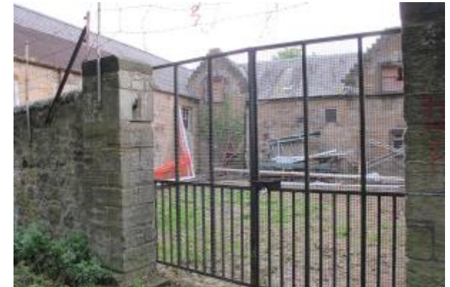
Current State of Stable Block
