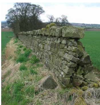
South park wall
