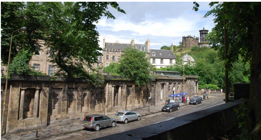
Screen wall of north section of the burying ground and the former Calton Convening Rooms seen from within the south section
