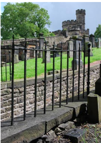
Original wrought iron railings, entrance to south section
