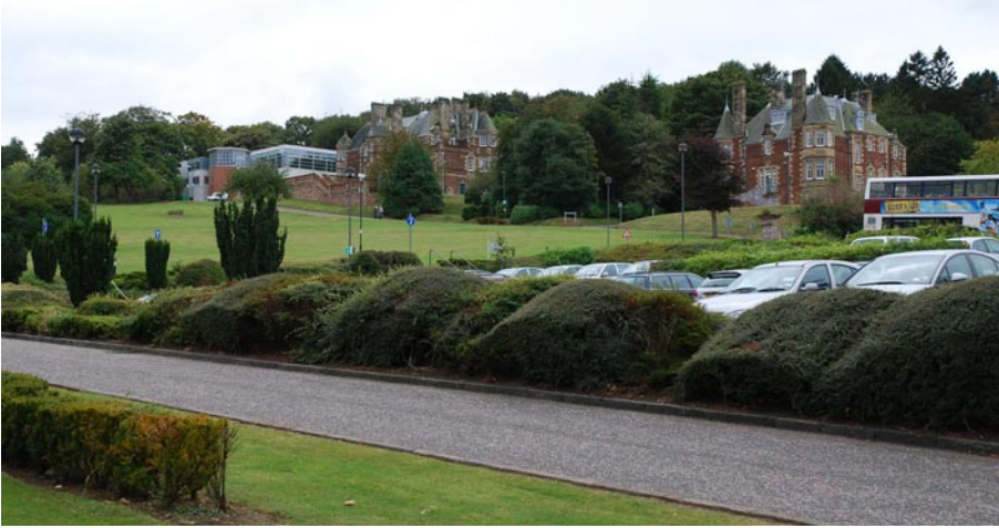
Main car park with LRC building, South Craig and Bevan villa in background
