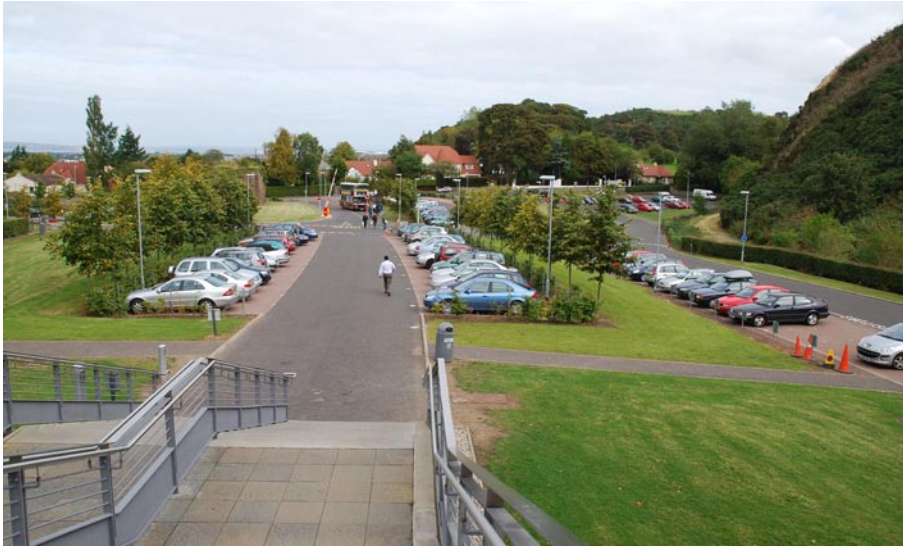
Approach to new building complex dominated by car parking
