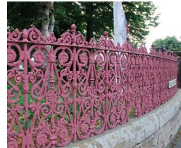
Railings at corner of Colinton Road and Glenlockhart Road
