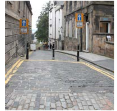
Overcomplicated road markings
