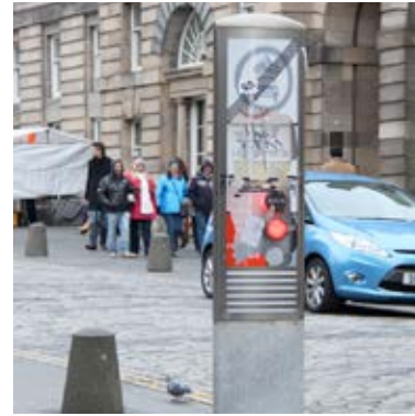
Damaged signage (this has since been fixed)
