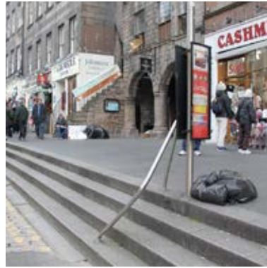
Damaged railings (now removed) and bin bags in the street
