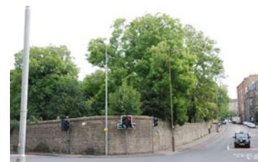
Cemetery wall at corner of Dalry Road and Henderson Terrace
