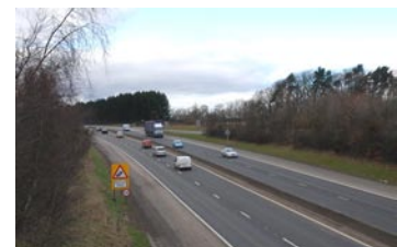
Bypass corridor from Dreghorn junction looking towards barracks
