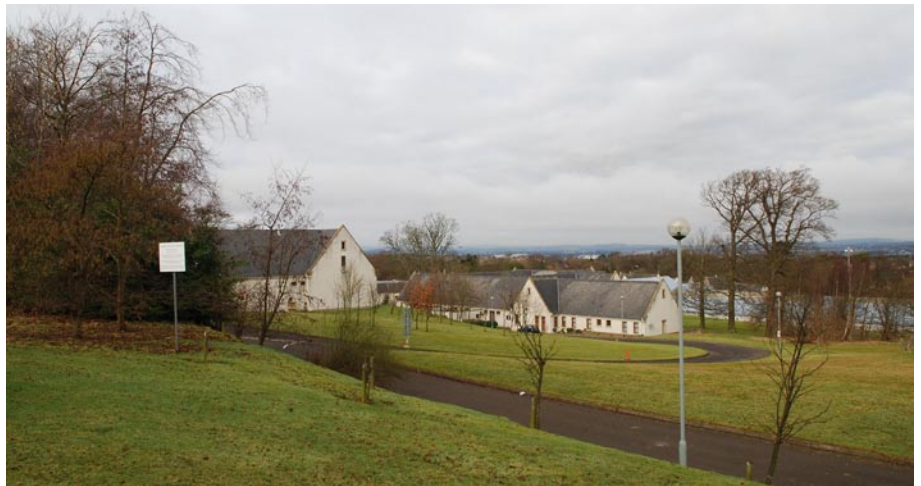
General view of the barracks from the south-east with distant view over Forth
