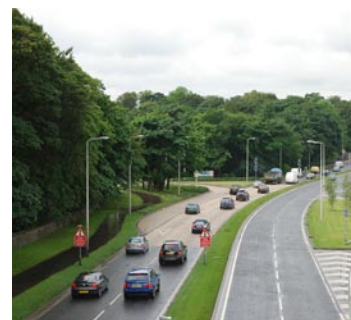
Boundary tree belt and main entrance area, Glasgow Road
