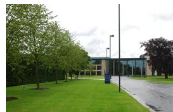
Road approach to main entrance
