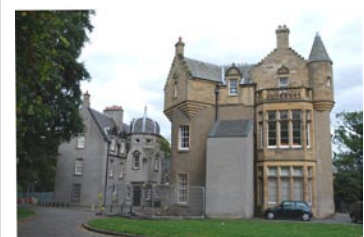
Inch House north-west end
