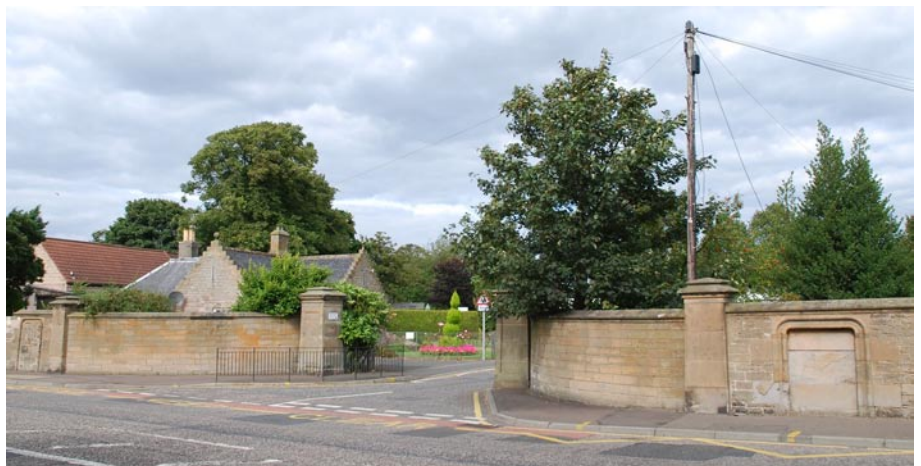
West gate and lodge, Gilmerton Road
