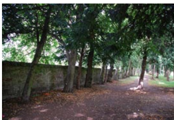
North boundary wall adjoining Cameron Toll
