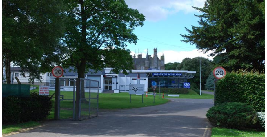
View towards house at stables entrance
