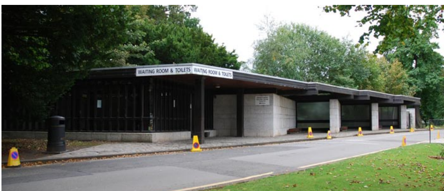
Waiting Room and toilets
