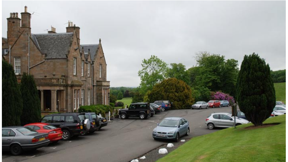
Norton House and south frontage
