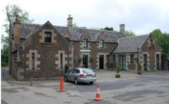
Stables block, conference centre
