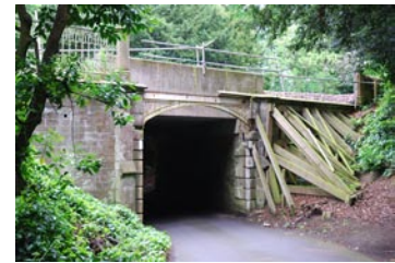
Railway bridge, North drive
