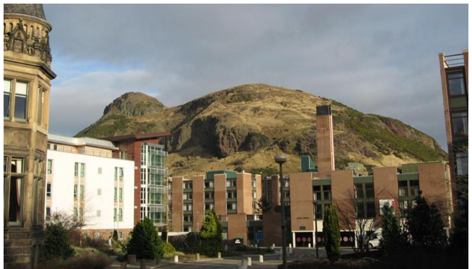
View in centre of Pollock Halls with three phases of built development and backdrop of Arthur's Seat
