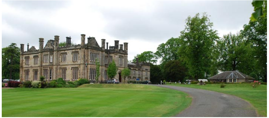
Ratho House (club house) with professional shop to right
