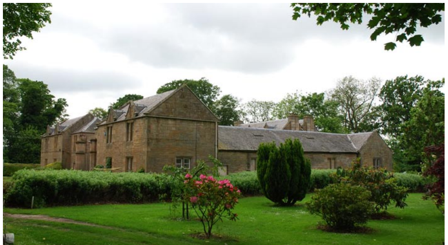
Stables courtyard from south-east
