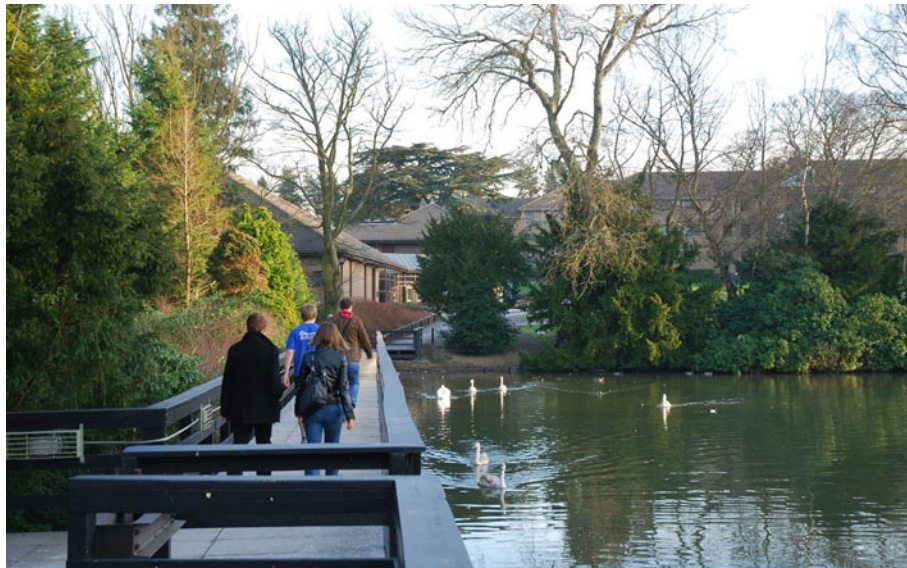
Walkway over loch dam
