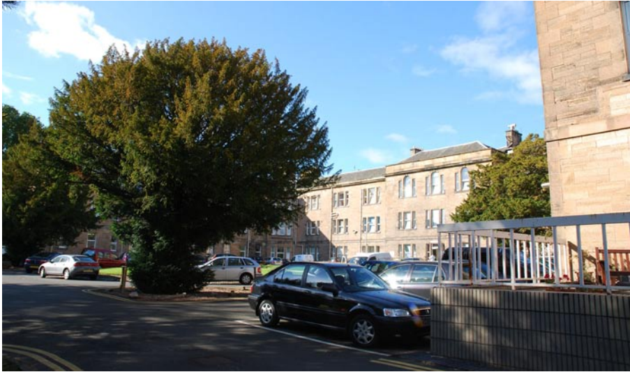
West House or MacKinnon House from south
