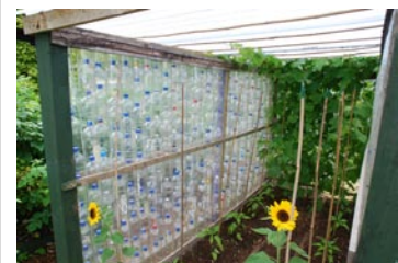
'Glasshouse' using recycled plastic bottles
