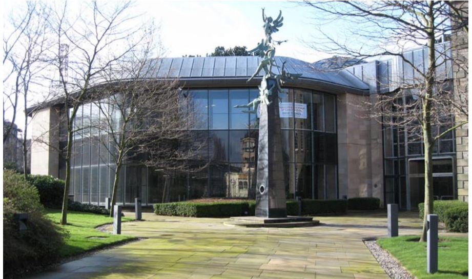
Tanfield House main entrance 2008
