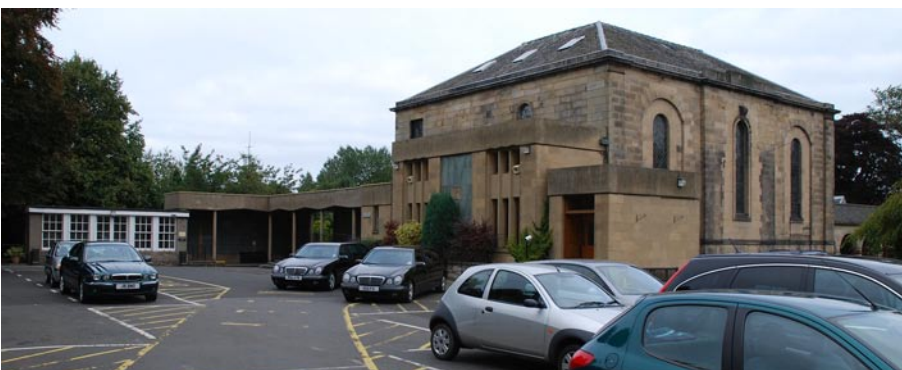
Entrance front and car parking, with waiting room in background
