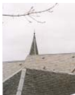
Traditional roof materials
