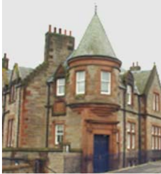
Former Paper Mill building
