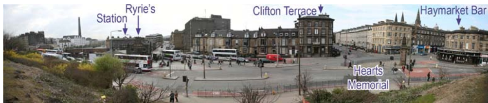
Photo 6 – View from Goods Yard
