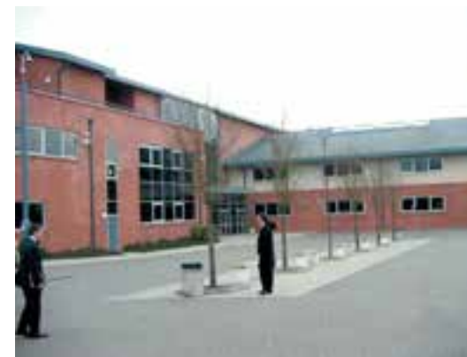
Balfour High School with Community Wing
