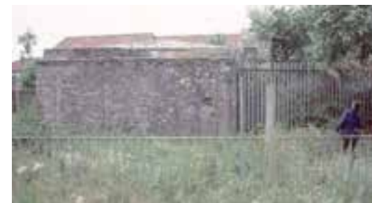
Niddrie Marischal Tombhouse - obscured and inaccessible
