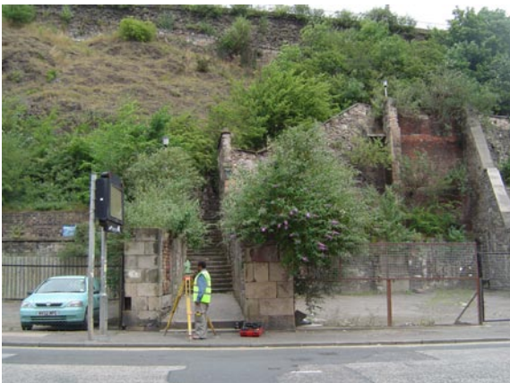
Figure 58: Existing steps to Regent road
