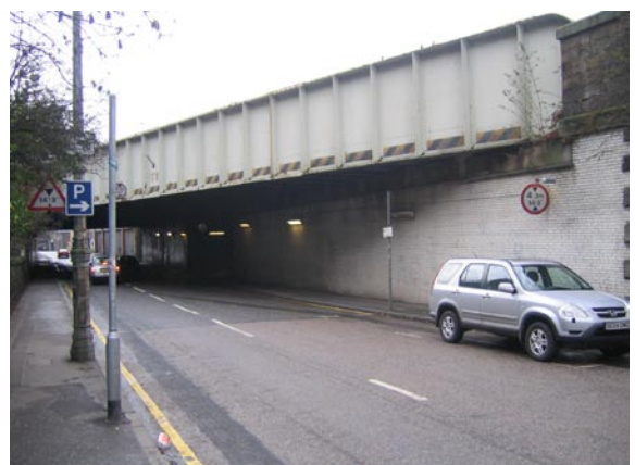
Figure 59: Railway bridge over Calton road
