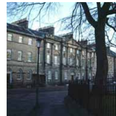
formal buildings fronting the square
