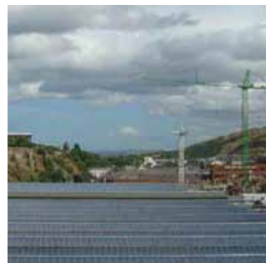
view east over the glass roof of Waverley
