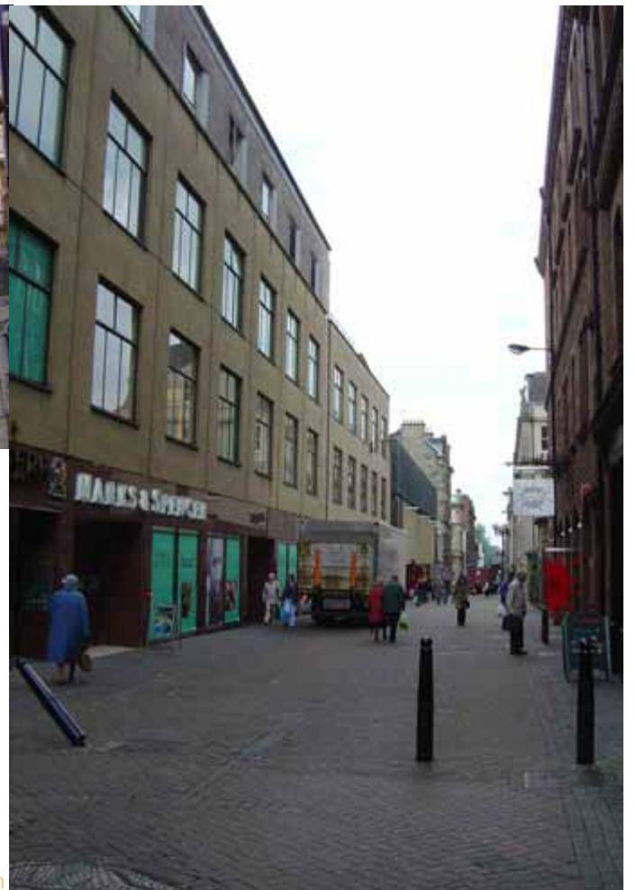
damage to public realm
