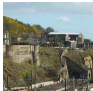
Old Royal High - rail tunnel below
