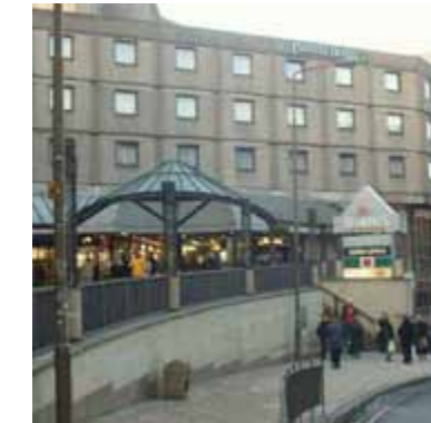
main existing entrance
