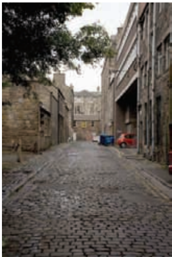
Rose Street Lane South, setted road and pavement surfaces with stone gutters (October 2007)
