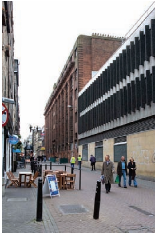
View G: along Rose Street west to east (Block 4 on the right)
