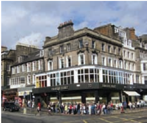
Previous tea room at first floor level
