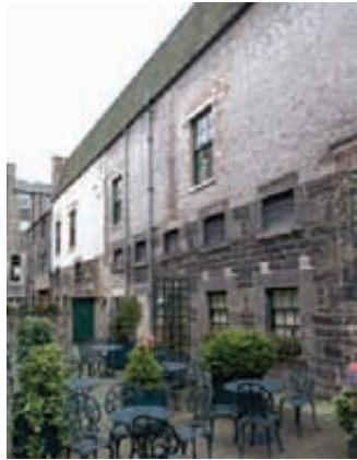
Mews buildings behind the south side of Charlottes Square (the five grouped openings relate to the original mews building for the central house)
