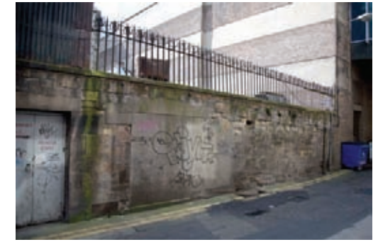
Garden wall behind No. 90 Princes Street. Blocked round-arched gateway in the centre (as depicted on Kirkwood's 1819 elevation); later railings.
