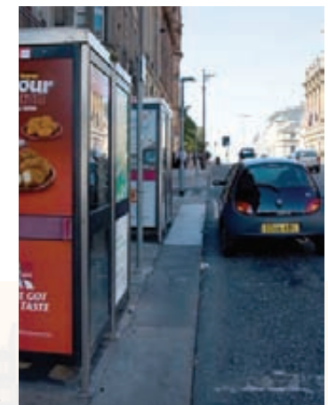
Run of substantial kerb stones in South St Andrew Street
