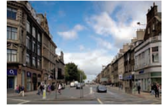
View F: south to north along South Charlotte Street
