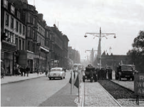
Removing the tram lines, 1952
