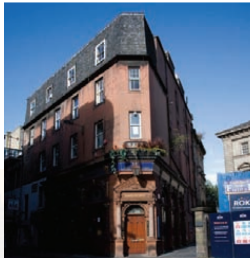
Guildford Arms, 3 West Register Street (September 2007) Tenement circa 1780. Ground floor altered in 1896. Roof also later.
