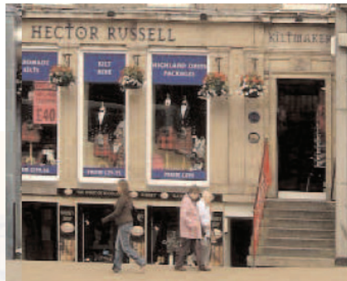
Surviving basement area
