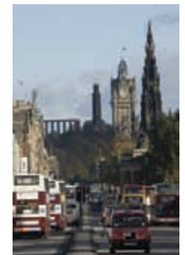
View east along Princes Street
