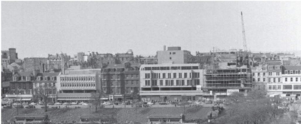
Work underway on the Panel building at Nos. 81-83 Princes Street, 1968
