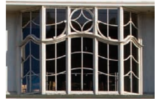
Nos. 119-120 Princes Street, window detail (August 2007)
