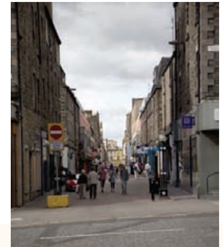
View G: along Rose Street east to west
