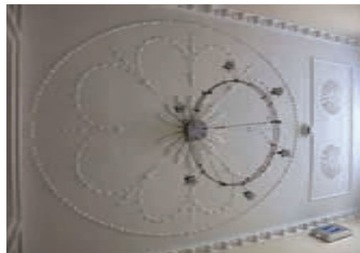
Fine late 18th century plasterwork in Castle Street
