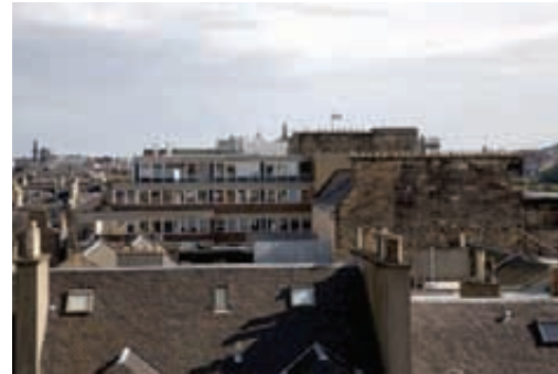
Roofscape of Block from South Charlotte Street (west to east). Tiered offices behind 124-125 Princes Street are in the centre of the photograph. (September 2007)
