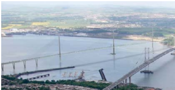
National development—Queensferry Crossing
