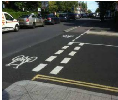
Transition across junction should be straightforward for users, and design – London Shoreham ( LCDS, 2016 ).
