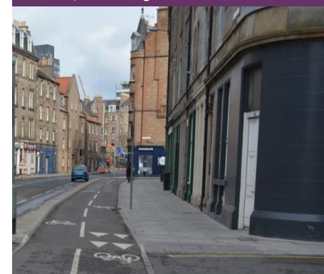
Hard surface buffer zone in Buccleuch Street, Edinburgh
