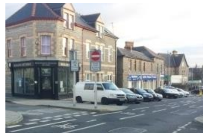
Contraflow cycling with advisory cycle lane, adjacent echelon parking with frequent cycle symbols, Penarth ( Sustrans Design Manual: Chapter 4 (2015) draft )
