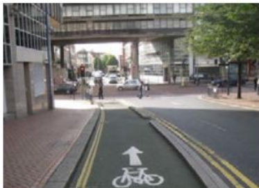
One-way contraflow cycle track on carriageway with curb separation, Hill Street, Birmingham ( Sustrans Design Manual: Chapter 4 (2015) draft )
