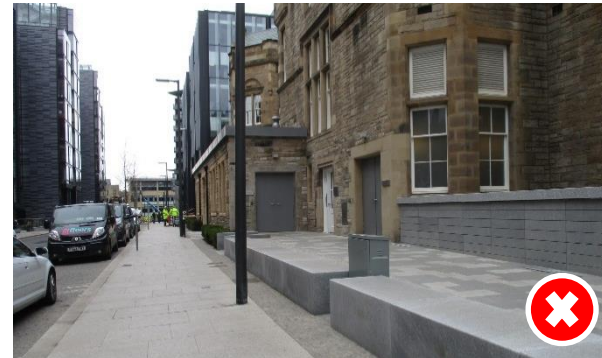
The City of Edinburgh Council: Poor positioning of street lighting, it could be placed further back in the footway so that it does not unnecessarily reduce the clear footway zone.
