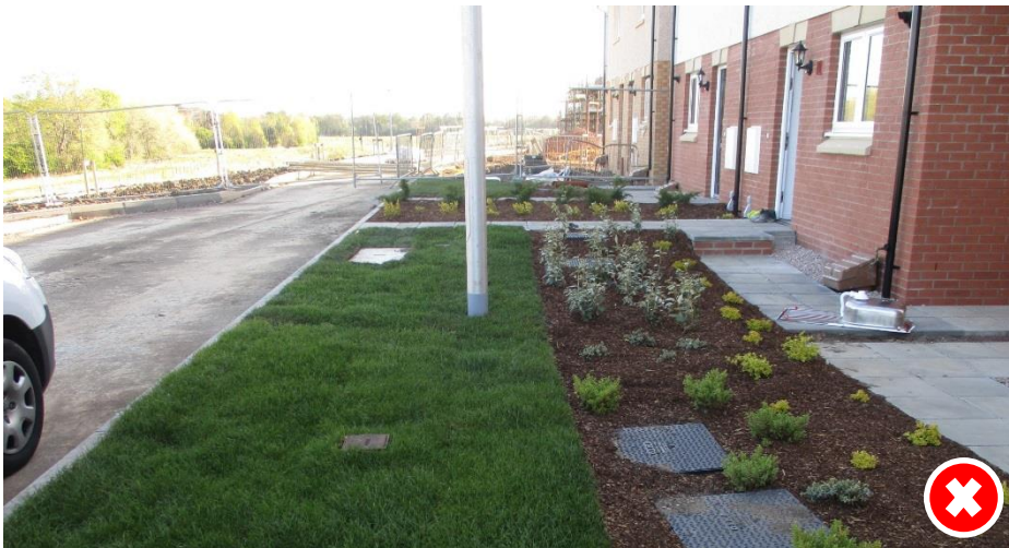
The City of Edinburgh Council: Poor positioning of street lighting, unclear to public/home owners whether the column is located in a service strip of front garden.
