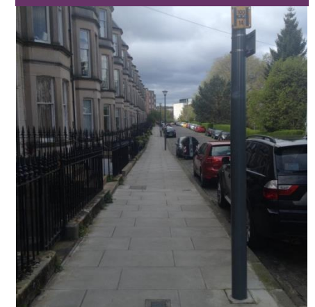
Street lighting located at the front of footway in conservation area
