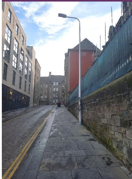
At back of footway on New Street
