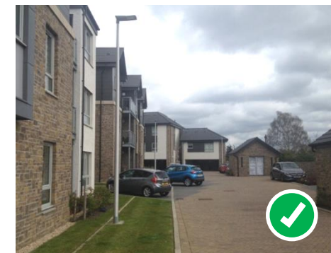
The City of Edinburgh Council: Good positioning with clear service strip area and demarcation line for ownership, also no tree/bushes planted near the columns.
