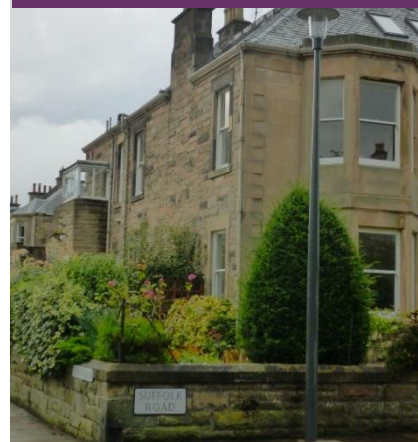
Street lighting located at the rear of footway in conservation area
