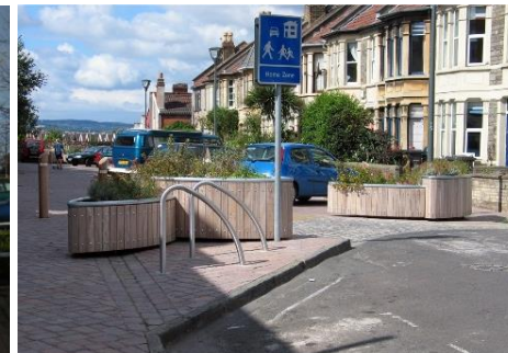
Transition points at road entry
