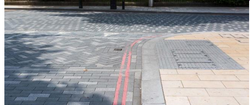
A raised table side road entry treatment in London
