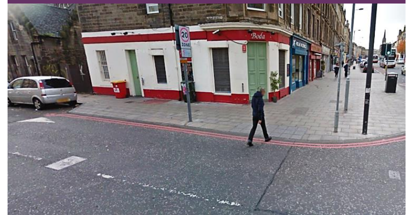
A side road build out on Lorne Street/Leith Walk, Edinburgh
