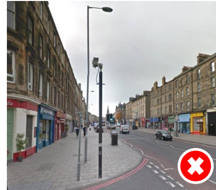
Google Earth 2017 : CCTV support placed next to lighting column and buildings, creating street clutter. Leith Walk, Edinburgh
