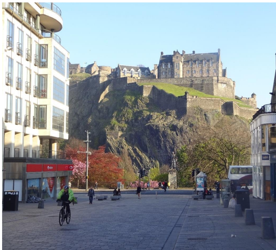
The City of Edinburgh Council: Successful application of de-cluttering on Castle Street to ensure the street acts as a stage for the wider urban realm.
