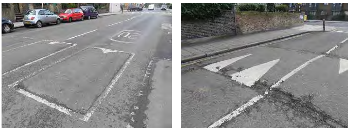
Photograph 2 (L-R): Speed cushions on Liverpool Road and speed hump on Furlong Road
