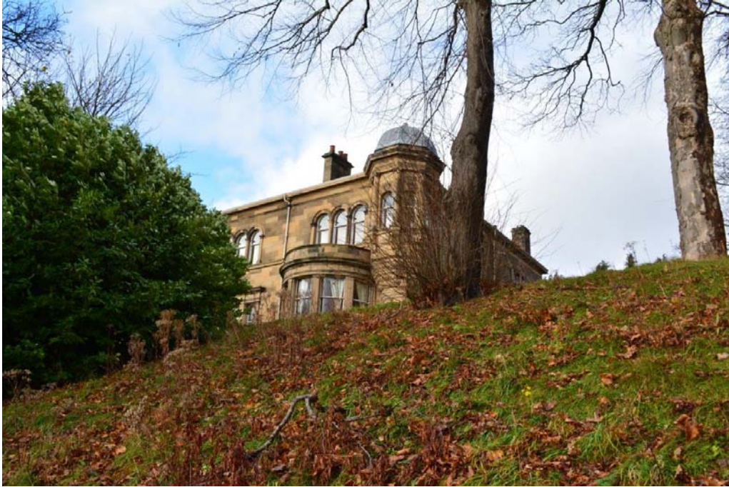
CAA 8 Beechmount House set on a small platform cut into steep wooded slopes
