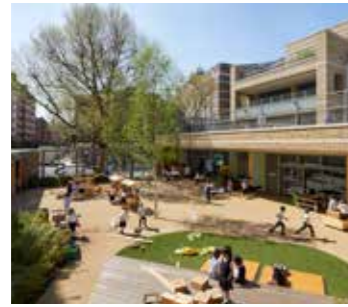
Fig. 3.15 Marlborough Primary School Client: Royal Borough of Kensington and Chelsea Architect: Dixon Jones Landscape Architect: Macgregor Smith Photographer: Paul Riddle
