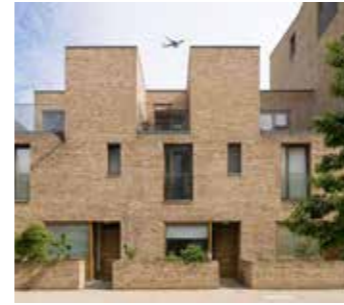
Fig. 3.52 Brentford Lock West Architect: Mikhail Riches Photographer: Mark Hadden & Tim Crocker
