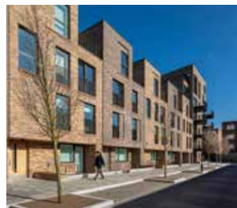
Fig. 6.5 Colville Estate, London Architect: Karusavic Carson, Photographer: © Peter Landers
