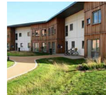
Fig. 3.18 E Image provided by LUC © 2B Landscape Consultancy Ltd https://www.2bconsultancy.co.uk/sustainable-drainage.htm
