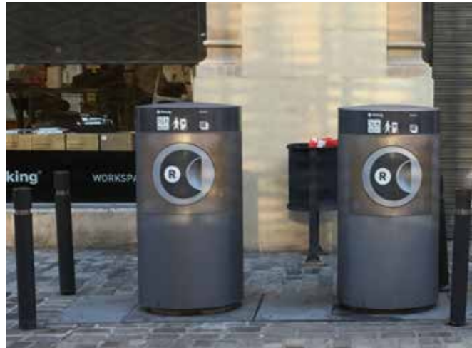
Fig. 3.71: Underground system in Barcelona
