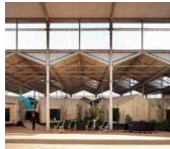
Fig. 3.66 A Red Bull Music Academy Architect: Langarita Navarro Arquitectos Photographer: Miguel de Guzmán
