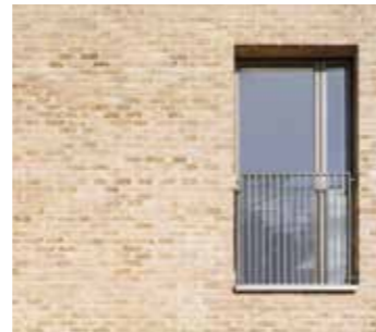
Fig. 6.23 b / 6.28 Brentford Lock West Architect: Mikhail Riches Photography: Mark Hadden & Tim Crocker
