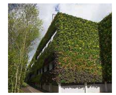
Fig. 3.19 A Image provided by LUC © One-world design architects http://www.one-worlddesign.co.uk/Project/national-grid-car-park
