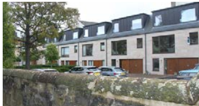
Existing stone wall retained with parking area behind results in minimal visual impact of parked cars at Malta Terrace
