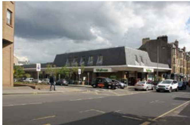
Rooftop car park for supermarket uses space efficiently and the building fully activates corner position along Morningside Road
