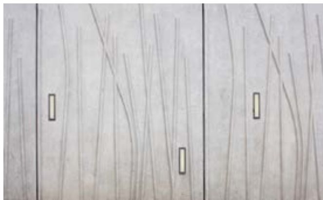
Concrete used sculpturally—Horse Wynd The sculptural potential of concrete is exploited in the Parliament wall with the patterned surface and integration of lights
