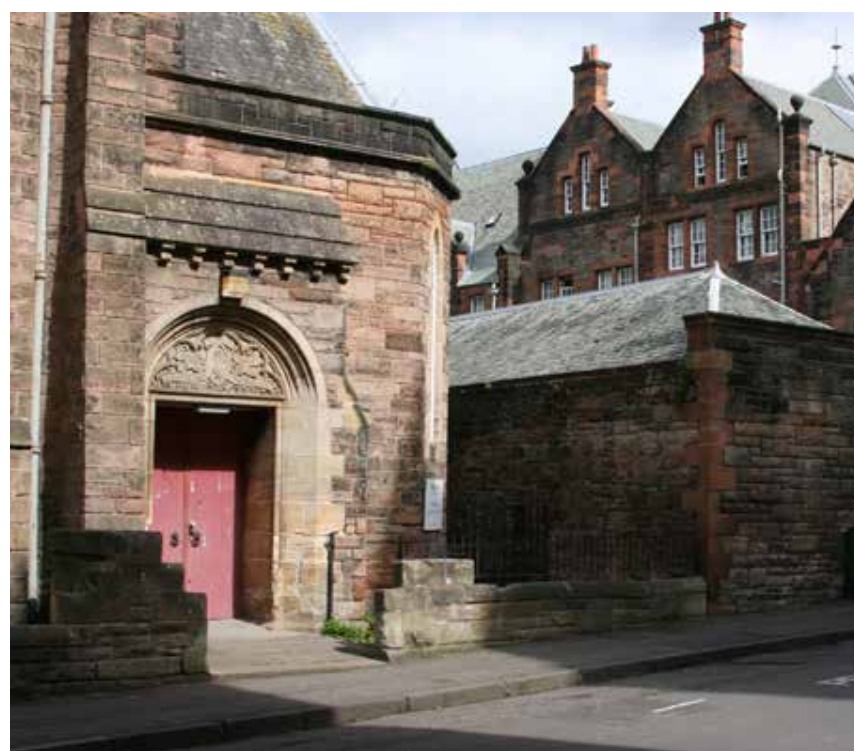
Montpelier level entrance
