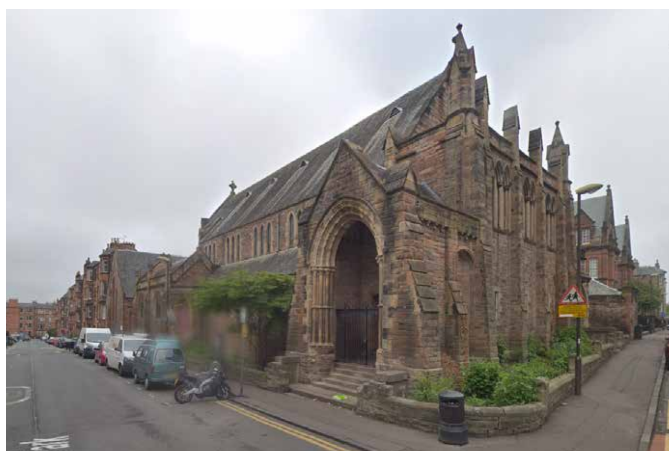
View from the corner of Montpelier Park and Montpelier
