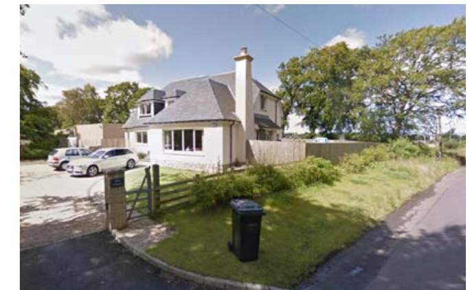
Existing house to south-east of site
