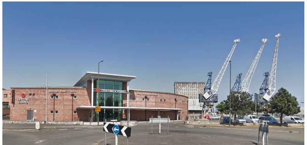
Figure 1: View of site from the South
