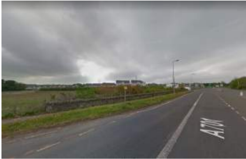
Street View looking North East
