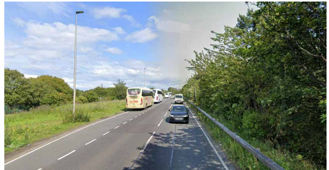
View along West Approach Road
