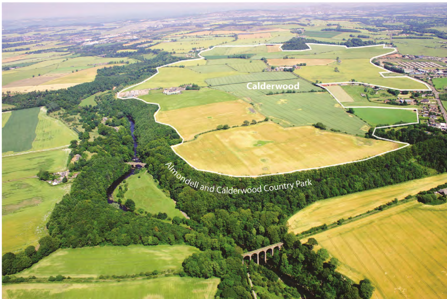
Before development, the 230 acre Country Park adjacent to Calderwood
