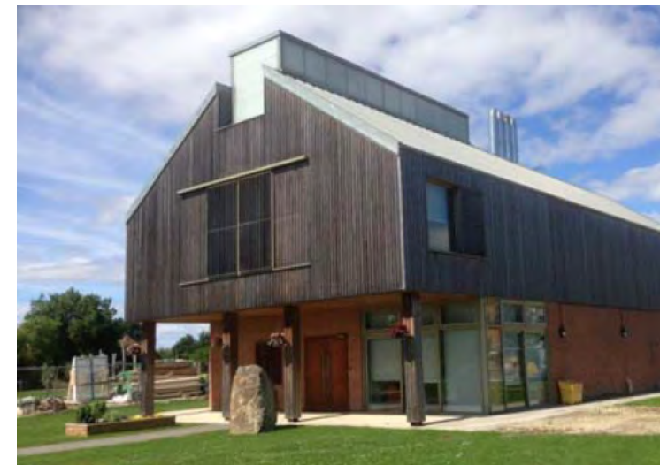
A centralised energy centre
