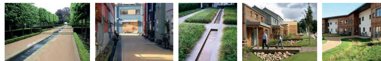
Fig. 3.18: Examples of blue-green infrastructure swales
