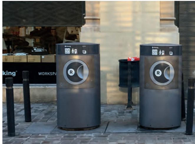
Fig. 3.71: Underground system in Barcelona
