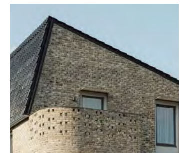
Fig. 6.12 Goldsmith Street Architect: Mikhail Riches Photo: ©Tim Crocker 2019
