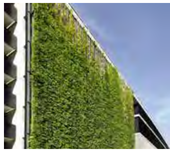
Fig. 3.19 B Image provided by LUC © One-world design architects http://www.one-worlddesign.co.uk/Project/national-grid-car-park
