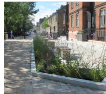
Fig 5.29 B Permeable paving and trench planter, London Image provided by AECOM
