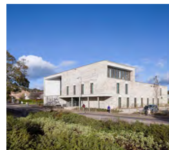
Fig. 3.66 H Allermuir Health Centre Architects: Hoskins Architects Photography: © dapple photography
