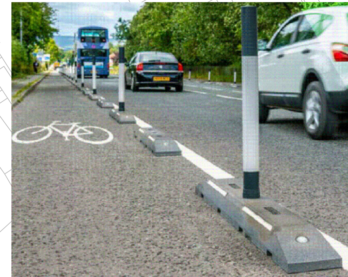
FIG 1. ROSEHILL NARROW CYCLE LANE DEFENDER UNITS - TO PROVIDE TRAFFIC SEGREGATION. PRODUCT 2.0M IN LENGTH & ARE BOLTED INTO CARRIAGEWAY WITH 5M GAP. NOTE CONTINUOUS WHITE LINING ON ROAD SIDE OF DEFENDER.
